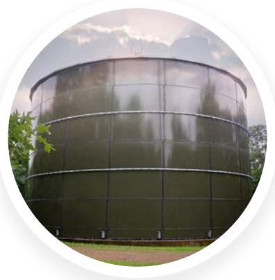
Ground Storage Tank
