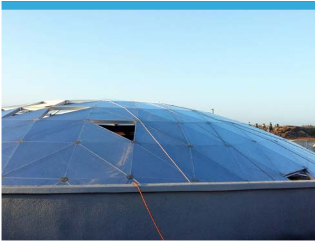
» Port Arthur Water Treatment Plant Port Arthur, Texas – 202' Diameter
