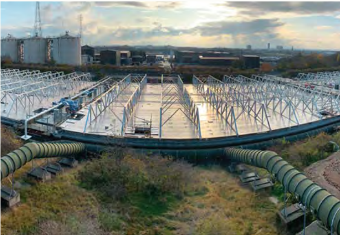
↑ Howdon Wastewater Treatment Works United Kingdom - Approx. 136,000 sq. ft.
