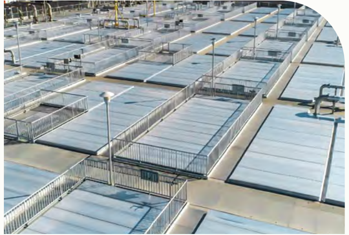
↑ Encina Wastewater Authority Carlsbad, CA - (8) 35' x 300'
