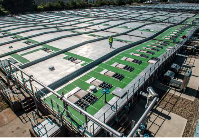
↑ Beckton Sewage Treatment Works United Kingdom - Approx. 600,000 sq. ft.
