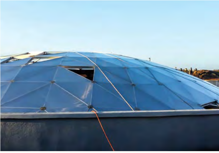
↑ Port Arthur Water Treatment Plant Port Arthur, TX - 202°
