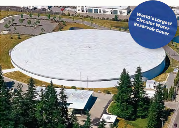
↑ Alderwood Water & Wastewater District Lynwood, WA - 375' Diameter
